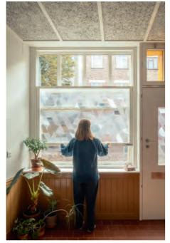
Above A secondary internal sash, fitted with obscured glass, allows privacy or visibility to the street.
